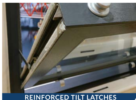
REINFORCED TILT LATCHES
